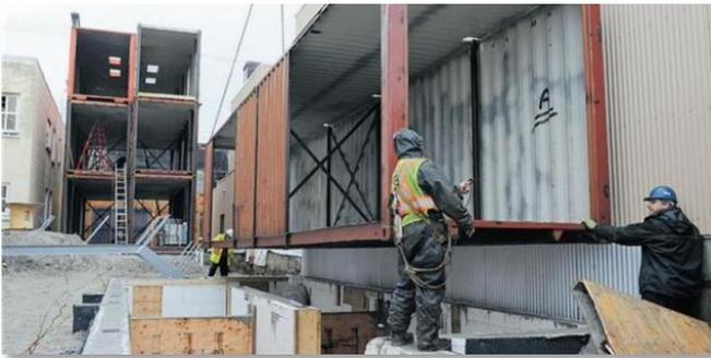
Twelve containers are dropped into place as construction begins on Canada's first multi-family recycled shipping container housing project. Photo by Jason Payne, *The Vancouver Sun*
